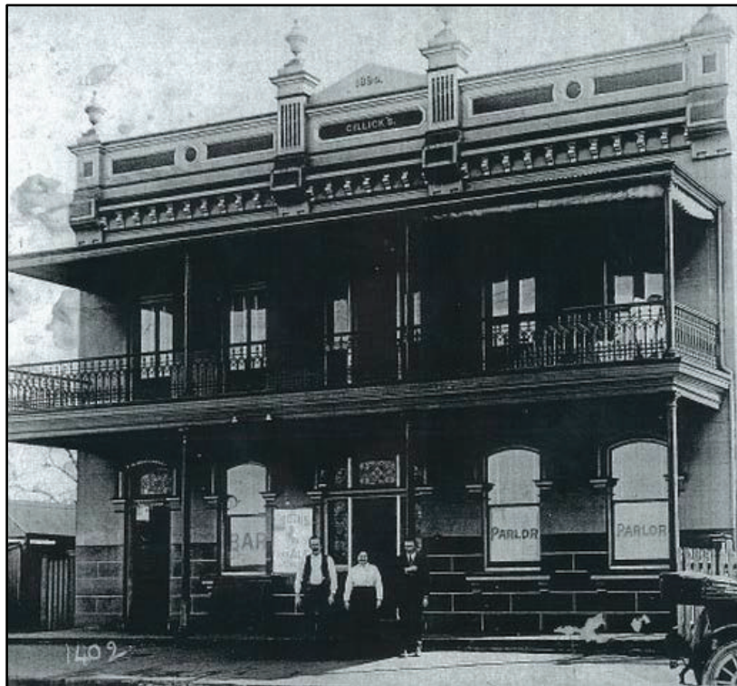
Figure 5: Photograph showing the Collingwood Hotel before its remodelling in the 1930s (Source: Collingwood Hotel website, History, available at: http://www.collingwoodhotel.com.au/index.php/home/history , accessed 04.12.14)
