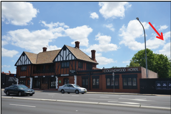
Figure 6: Primary façade of heritage item Collingwood Inn Hotel located in the vicinity of the subject site (the latter’s approximate location is indicated by the red arrow) (Source: Rappoport Pty Ltd, taken in 28.11.14)
